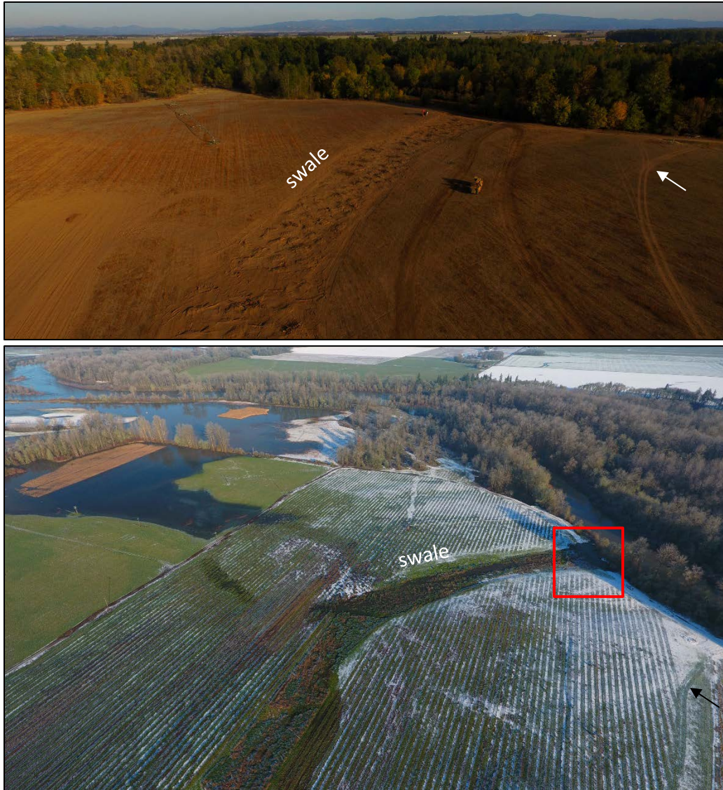
Figure 3-1. Example of floodplain swale restoration from Harkens Lake on the Willamette River. The project swale is labeled, and black and white arrows mark same location on road for reference. Top: Recently completed construction floodplain swale construction. Large wood elements are visible in the swale. Bottom: View of same swale the following winter showing inundated conditions. Red box marks location of low water gravel crossing pictured in Figure 3-4.
