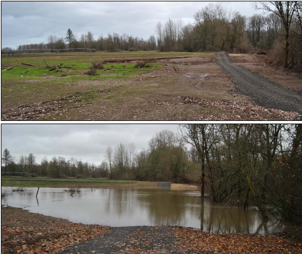
Figure 3-4. Example lower water gravel road crossing from the Harkens Lake pictured in Figure 3-1 showing dry (top) and inundated (bottom) conditions. Typical design large wood elements are visible in both photos.
