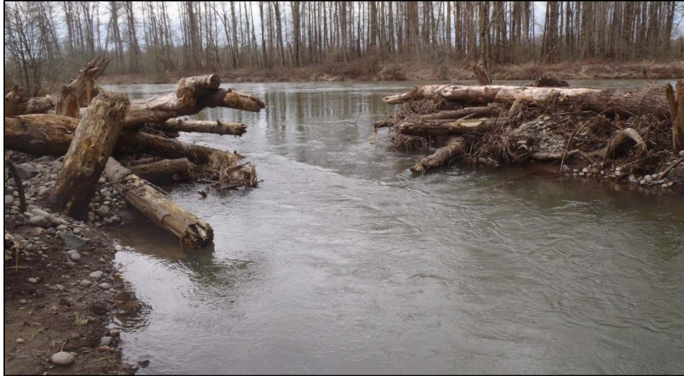
Figure 3-3. Example of the use of large wood stabilization measures at a side channel inlet from Green Island on the Willamette River. View is towards mainstem Willamette from the side channel.
