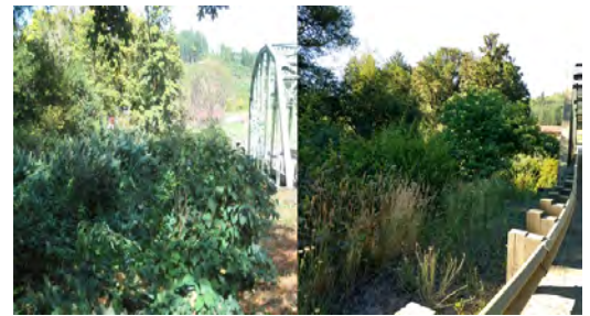
Wildwood Bridge before and after knotweed control treatment.
